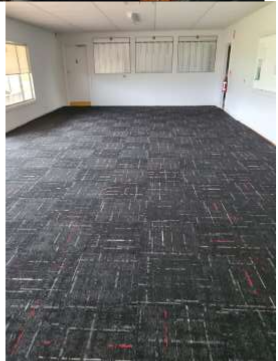
Carpet upgrade is underway at the club house
